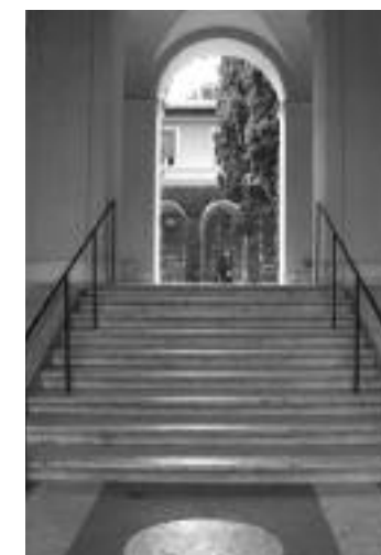
Steps leading into the AAR courtyard
